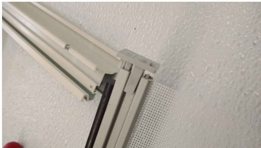
You are ready to put the blind back together. When sliding corner into siderail make sure the radius slides into notch. It is easiest to do this first to both ends before pushing below the notch to click it in place
