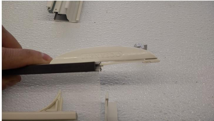
Slide new handle the exact way you took it off old one through notch in xbar. When it hits the nib push in and slide the rest of the way
