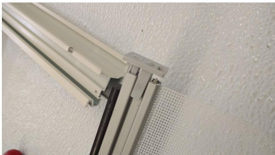
You are ready to put the blind back together. Make sure blind/screen is rolled tightly. When sliding corner into siderail make sure the radius slides into notch. It is easiest to do this first to both ends before pushing below the notch to click it in place
