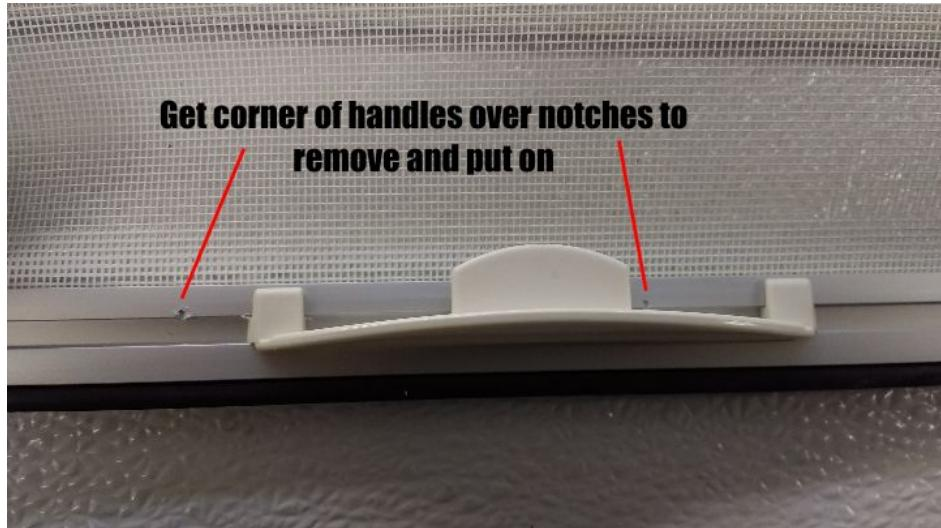
Get corner of handles over notches to remove and put on
