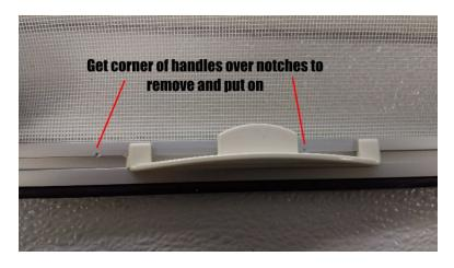
Slide off handle. BE AWARE WHAT WAY HANDLE IS FACING. Slide new handle the exact way you took off old one through notch in crossbar. Use soft tip hammer to bump handle over notches in crossbar
